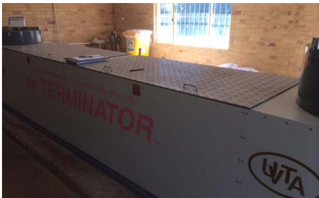
UV radiation acts as a tertiary treatment to disinfect the water.
