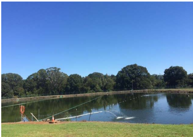
Balancing ponds store the water before being reused for irrigation purposes.
